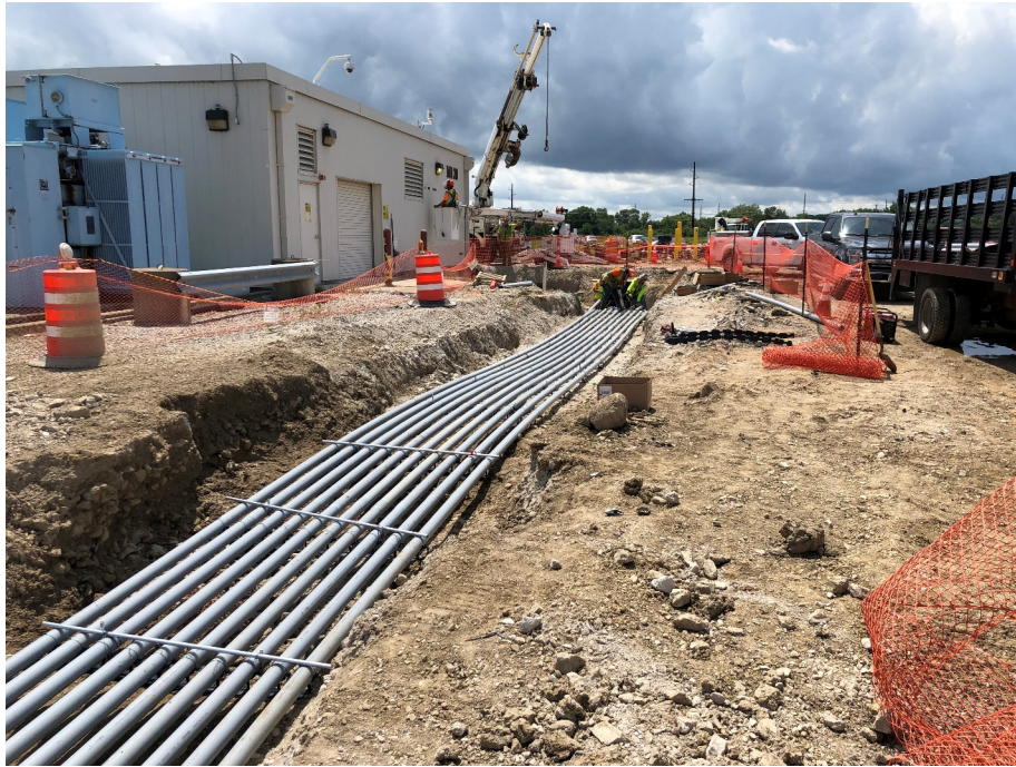
Installation of new power and communications duct bank
