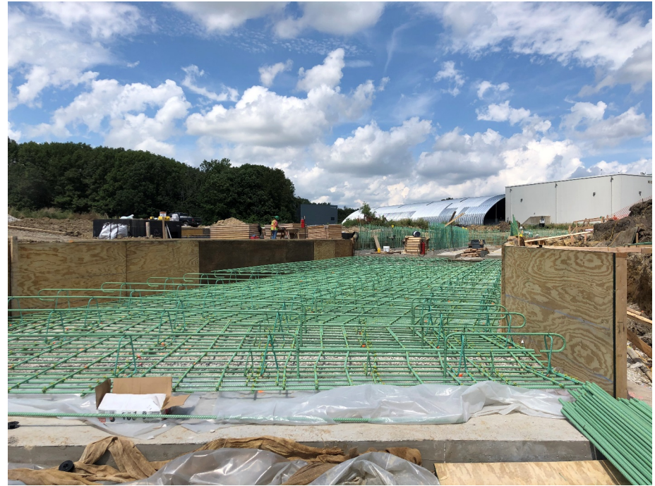
Installation of Indian Creek culvert reroute
