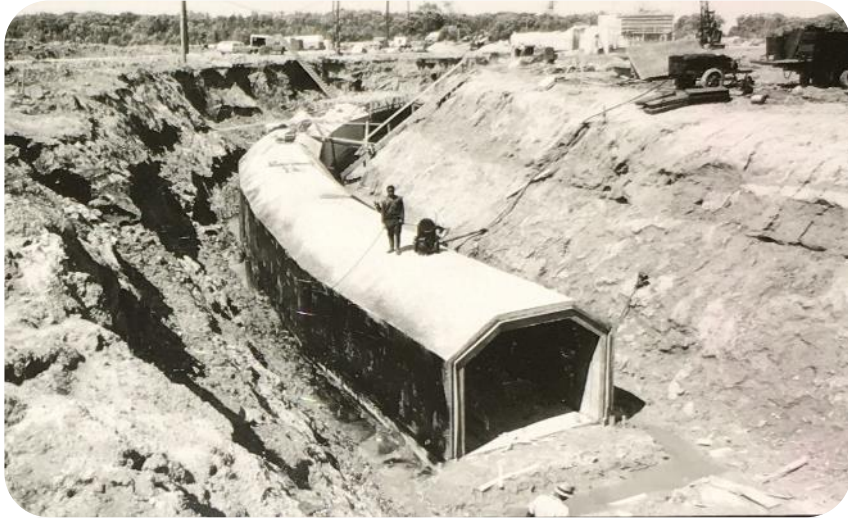
Tunnel forming and sealing of exterior. 1969
