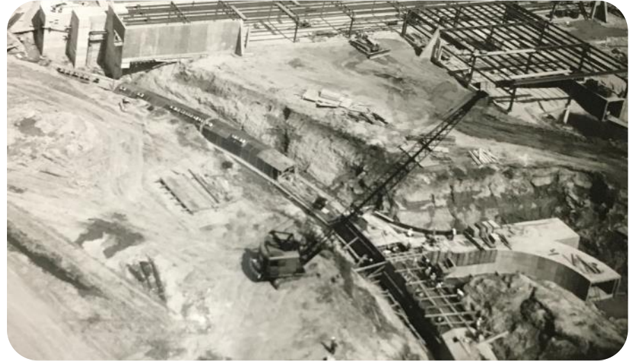
Tunnel sections being formed 1969
