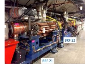
Solid state driver in gallery connects to PA amp in tunnel. Improved PA lifetimes and
