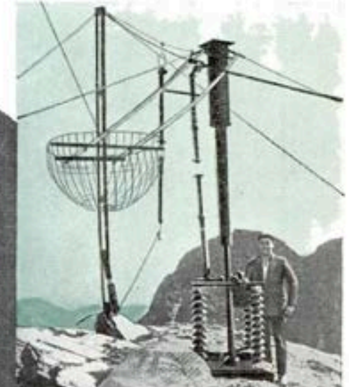
Here is part of the apparatus that was used in the Mt. Generoso tests. This strange network was designed to carry the enormous voltage to the laboratory where the scientists waited in danger of instant death.
