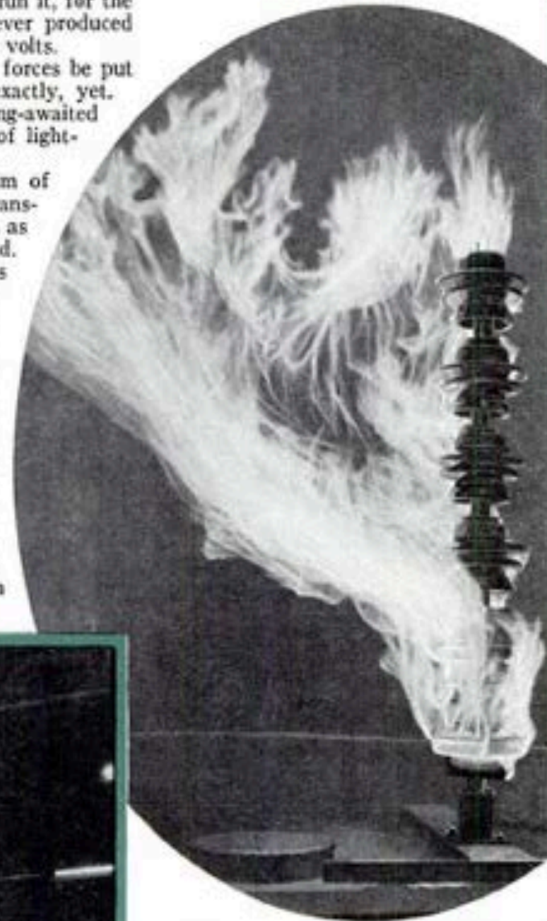
This is not lightning, but a discharge of laboratory electricity leaping from insulators. It shows why extraordinary apparatus is required in harnessing 18,000,000 volts.
