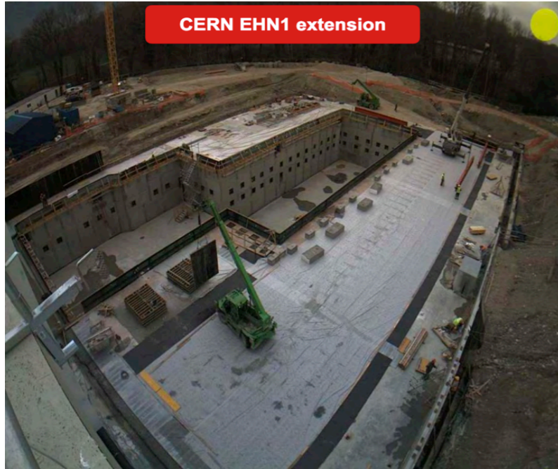
March 2016, construction of EHN1 extension
