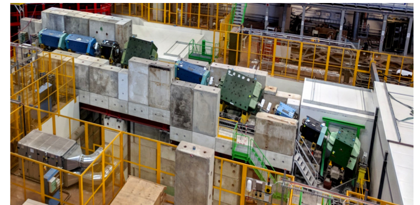
September 19, 2018 - ready for beam!
