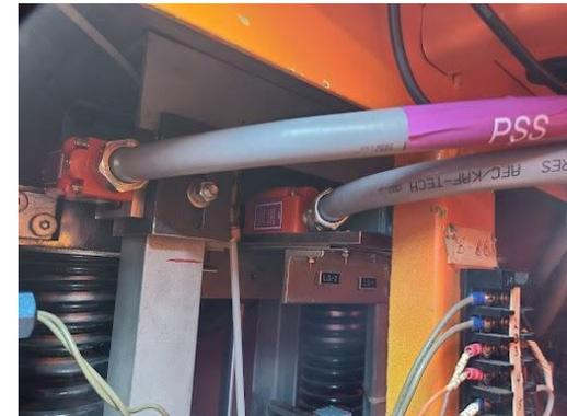
PSS-SIS Position Sensing Switches on Coil High Current Switch
