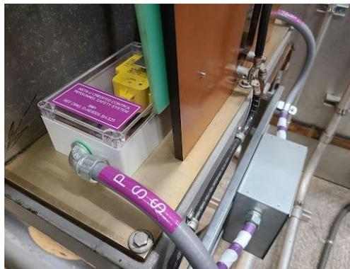
PSS-SIS Position Sensing Switches on Neutral Beam Ground Switch
